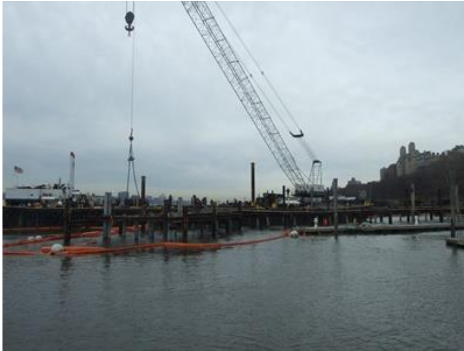
A Dock construction – December, 2015
